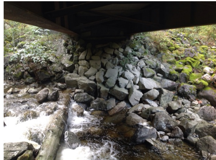
Left Bank Abutment when facing downstream
