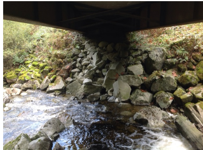
Right Bank Abutment when facing downstream
