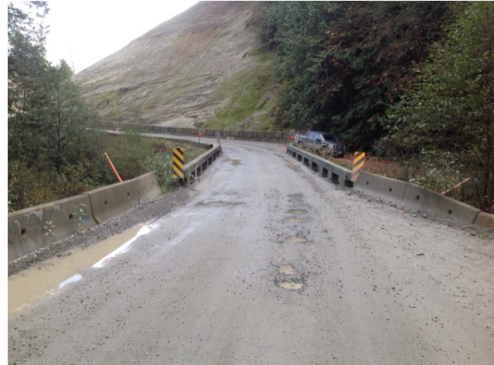
Approach from Left Bank when facing downstream
